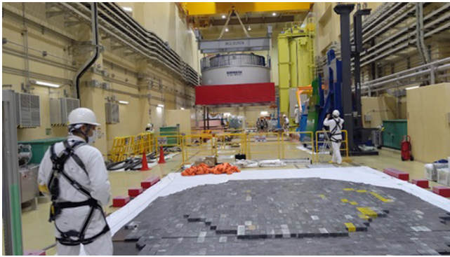
Fig. 3. Gamma-ray shielding layers consisting of iron plates and lead blocks. The 70 tonne detector with Gd-LS and LS was transported by a crane and installed on the shielding layers.
